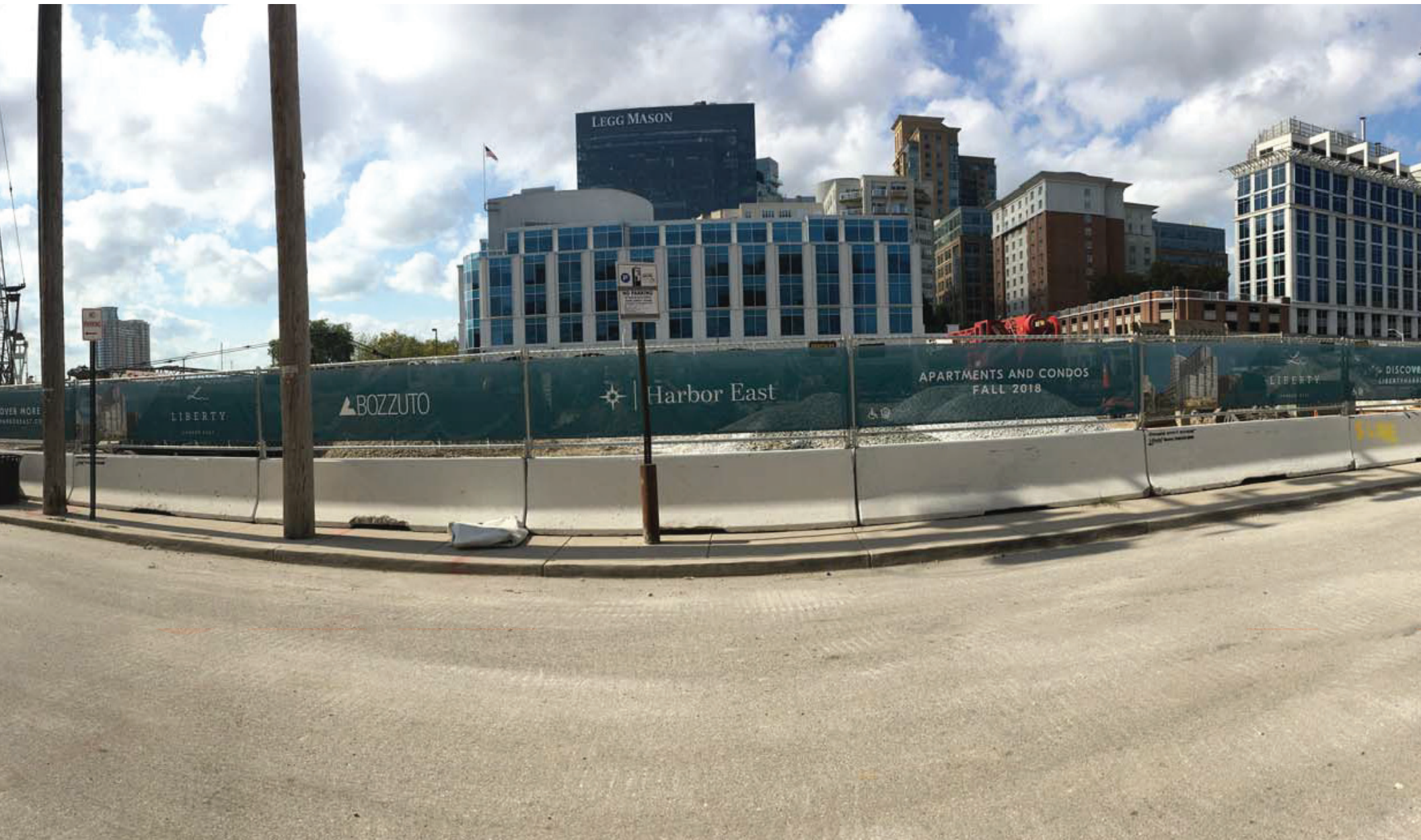
Sample Chain Link Fencing with Decorative Wind Screening and Jersey Barriers
